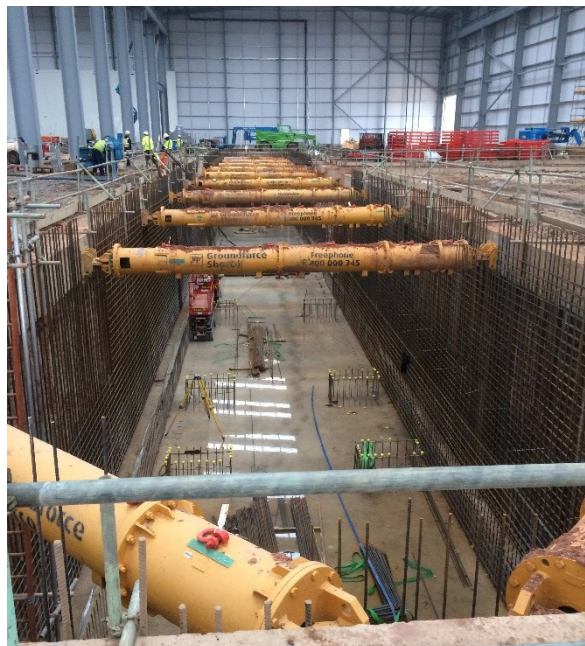
Figure 3: Seven metre deep press pit construction in manufacturing facility required the use of FLI QDS' water management expertise
